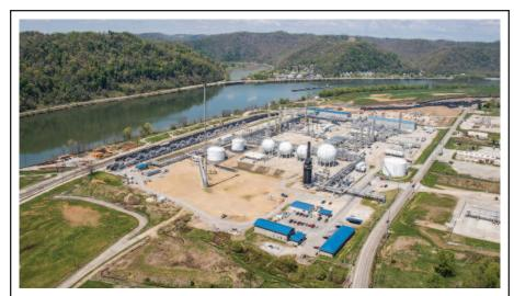
Blue Racer Midstream's Natrium natural gas processing and fractionation facility, which is located on the Ohio River in Marshall County, W.V., has a processing capacity of 400 million cubic feet of natural gas a day. The facility's 123,000 bbl/d fractionator strips the ethane, propane, butane, propane and natural gasoline from the Y-grade natural gas stream fed into the plant.
